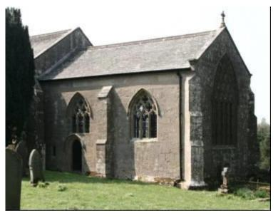
pointed arch of two continuous orders, the outer with a hollow chamfer, the inner a straight one, under a simple moulded hood with carved stops. Each bay has a window of three ogee-headed cusped lights with reticulated tracery that seems all restoration, within an old chamfered frame and moulded hood with carved stops; the sill of the western is set higher, to clear the priest's door below.
