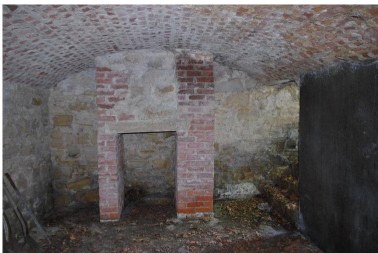
The vault, looking west, showing structure of uncertain function
