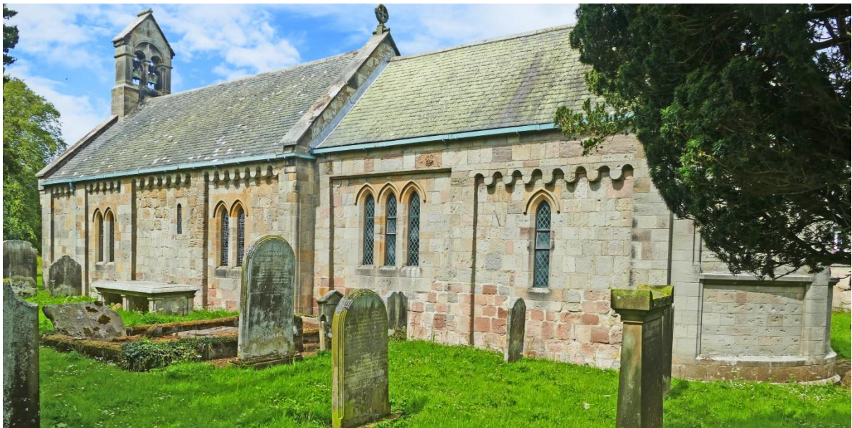
The church from the south east
