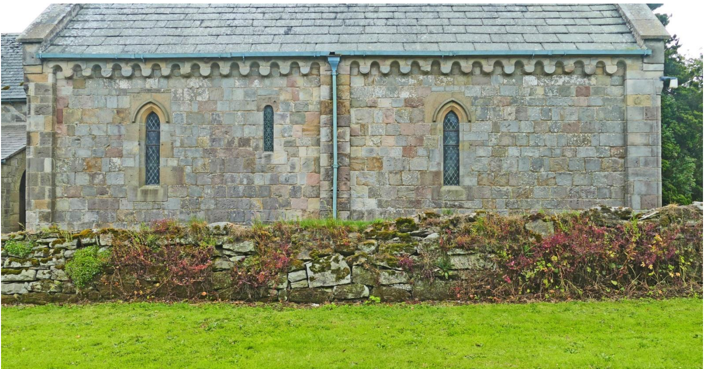
North side of north aisle, originally north wall of nave rebuilt in new position in 1866
