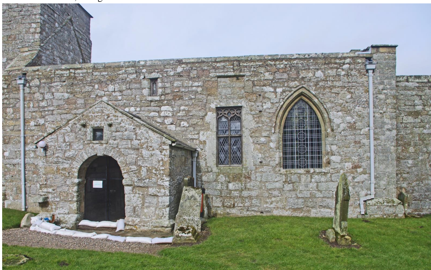
The Nave from the south
