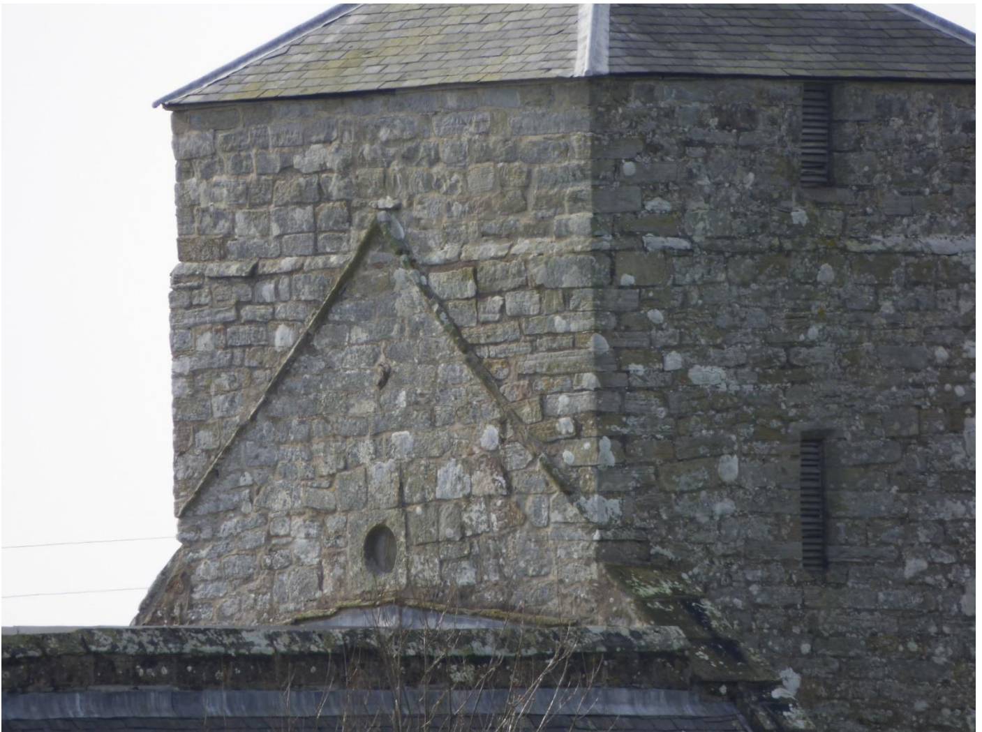
The east side of the tower, showing the roof tabling of the early gable and the internal face of the oculus
